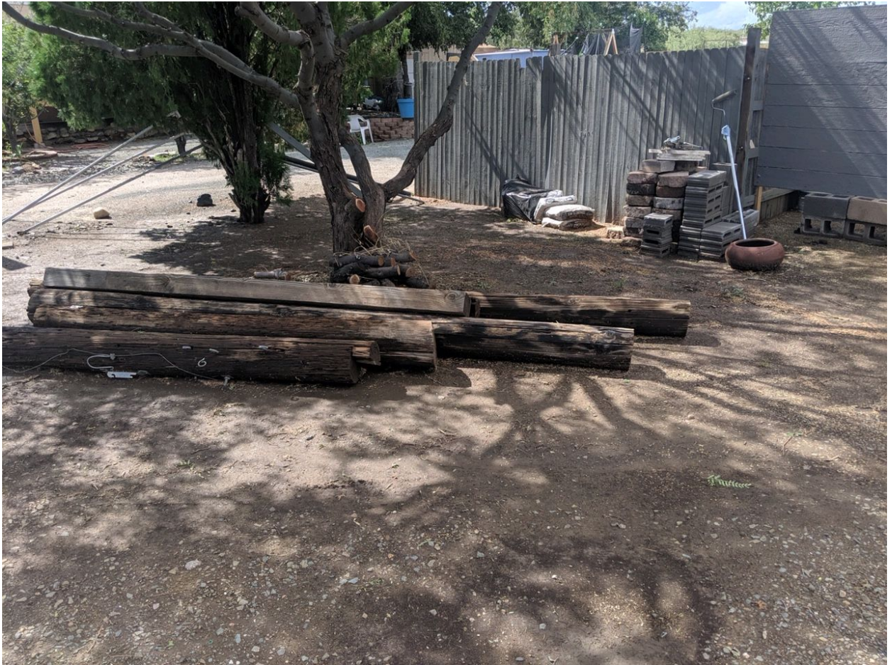
Image E - Storm Damage
